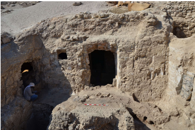
Fig. 14. The facade of MIDAN.05 with the original window, later closed. The closure mud bricks are still visible in the lower part. @MIDAN.05
